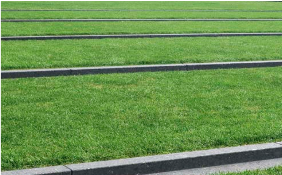
Low Retaining Walls
