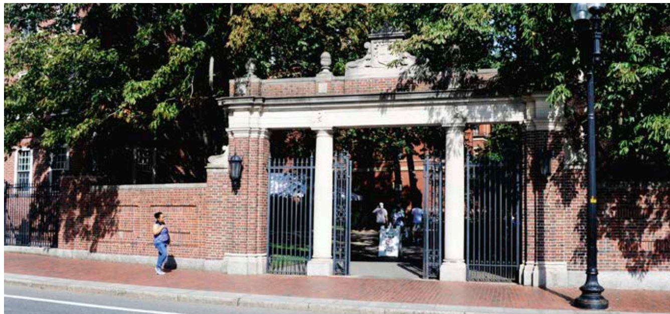
South Eastern boarder of Harvard Yard
